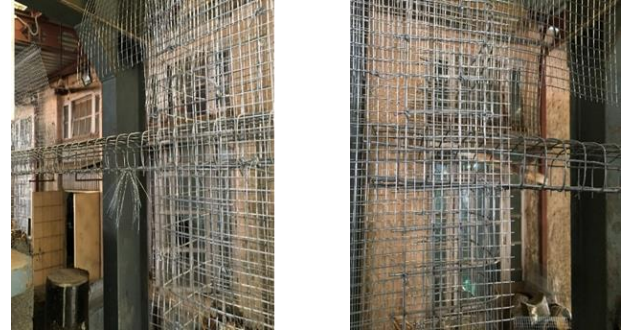
Fig.2 (b) provision of lintel at the opening
