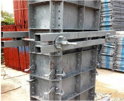
Figure 4: Steel Formwork
