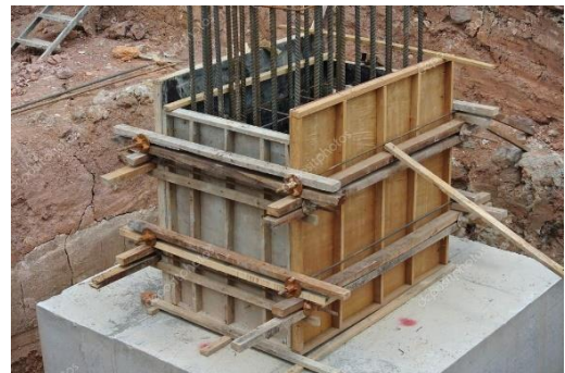
Figure 3: Plywood in combination with timber formwork
