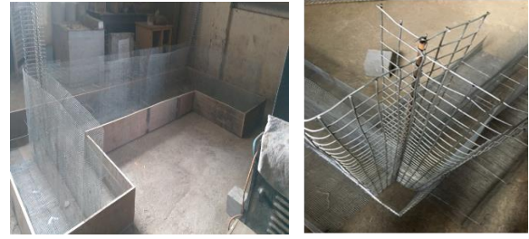
Fig.2 (a) Formwork for foundation and details of wall-to-wall connection
