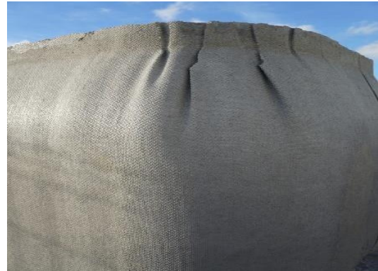
Figure 7: Fabric Formwork
