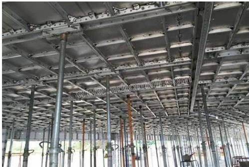
Figure 5: Aluminum Formwork
