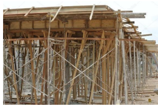
Figure 2: Timber Formwork
