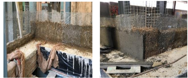
Fig.2 (c) Earth and straw filling, compacting and plastering of
